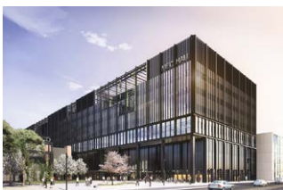
Manchester Engineering Campus Development, UK
